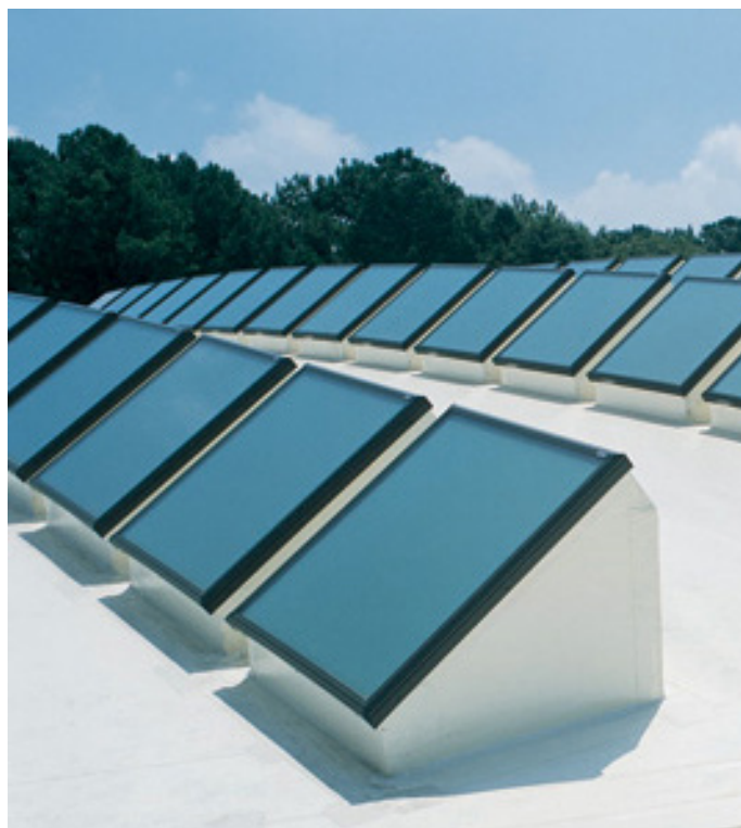
Fig. 10. Illustration of curb-mounted skylight arrays. (Note: not actual installation on this project)
