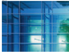
TRANSPARENCY, OPENESS AND DAYLIGHT: CLEAR, TINTED AND SPANDREL GLAZING IN ALUMINUM FRAME
