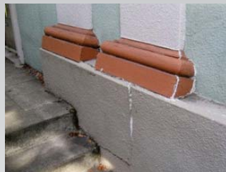
Dry-rot and termites in cripple wall; cripple wall not salvageable; exterior walls require seismic strengthening
