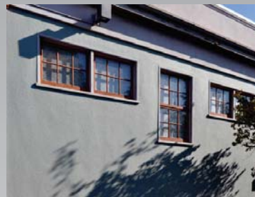
Head, jamb and sill extensions required; Fungal infection in some areas; Single-glazing
