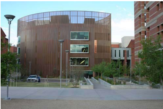
CURVED WOOD WALL
