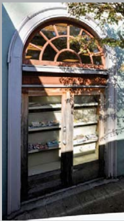
Door is not original design or construction; single-glazed window
