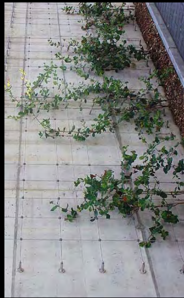
Concrete wall with cable trellis
