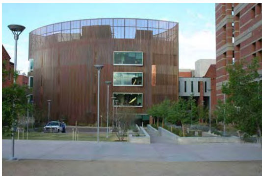
CURVED WOOD WALL
