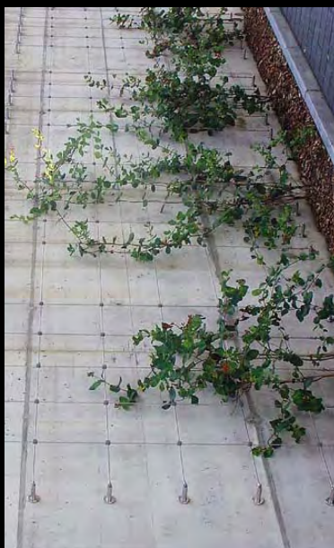
Concrete wall with cable trellis
